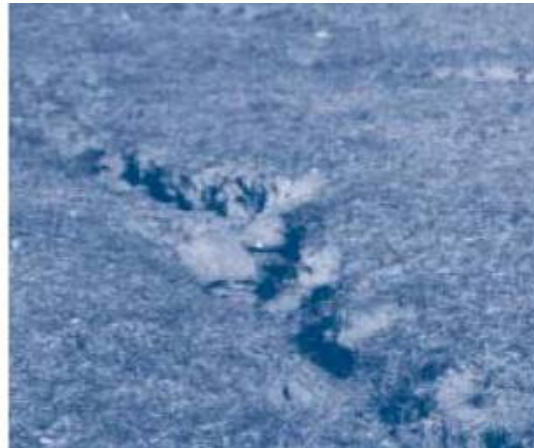
Figure 4.2 Large fissure in a landfill cap (>3 cm wide)
