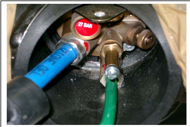
Electric Valve with Supplementary Manual Screw:
