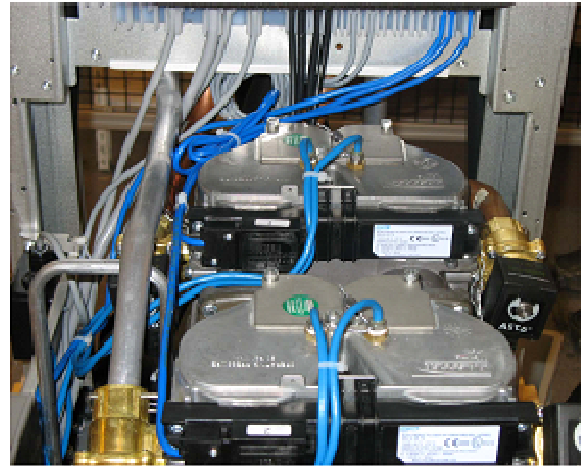
Figure 34 Probes mounted in dome cover
