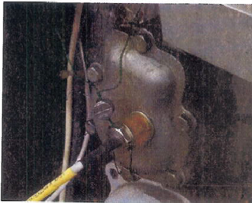
Figure 7 Sealing of temperature probe
