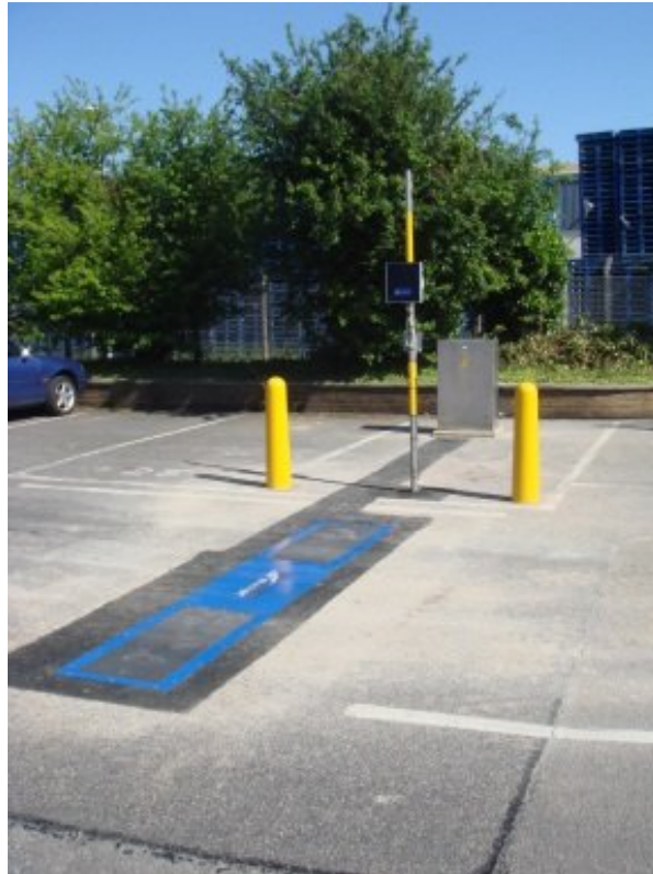
Figure 4 Typical Installation of the weighing system
