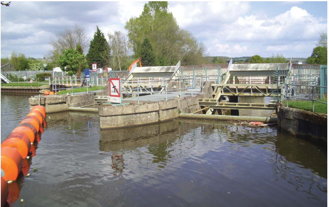
↑ Sluice gates at the Yalding Depot.
