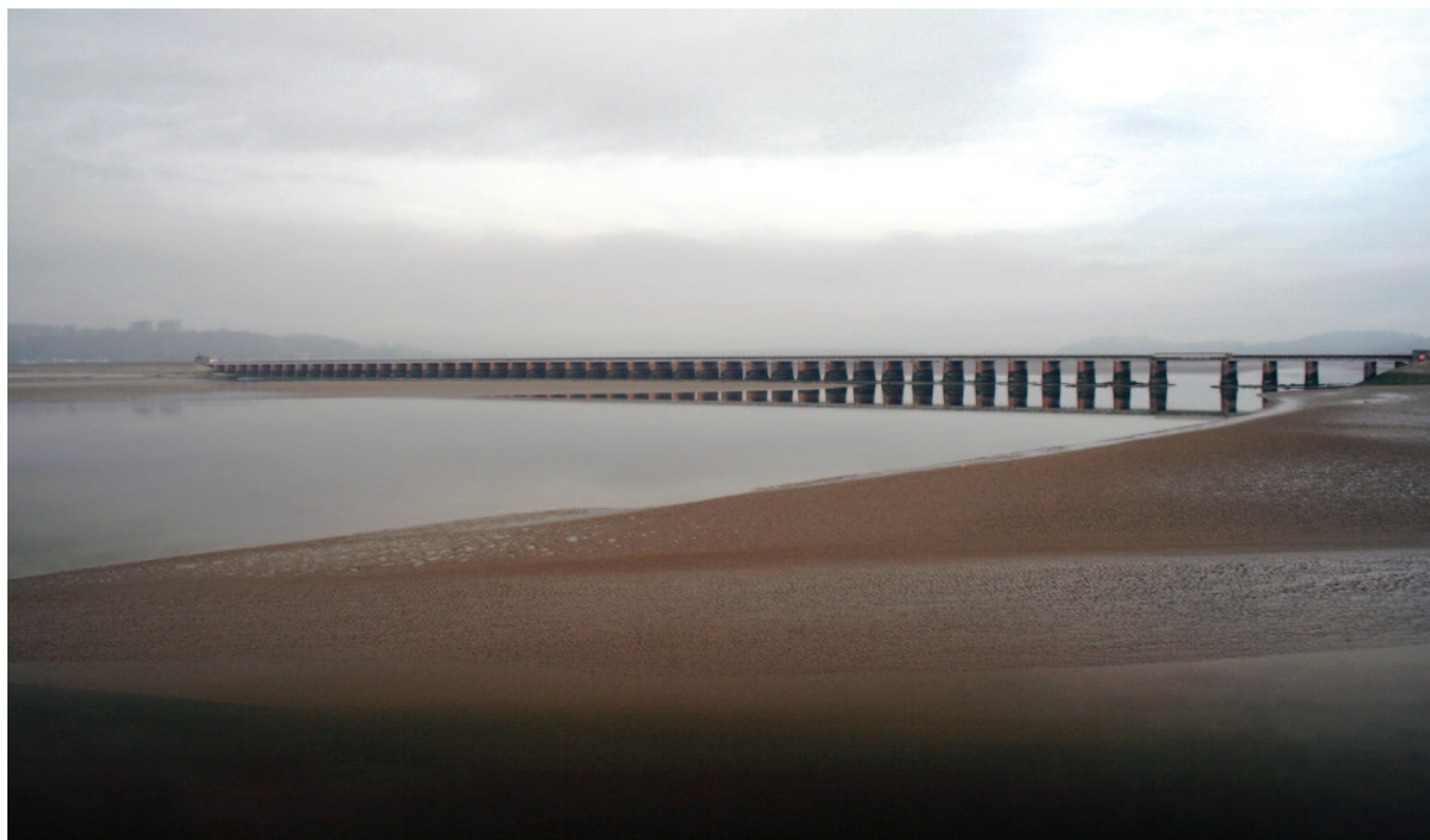
↑ The Kent Viaduct from Arnside
