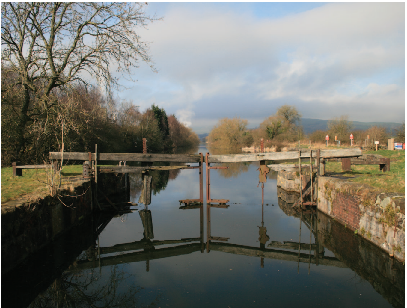
↑ Obsolete lock at Canal Foot
