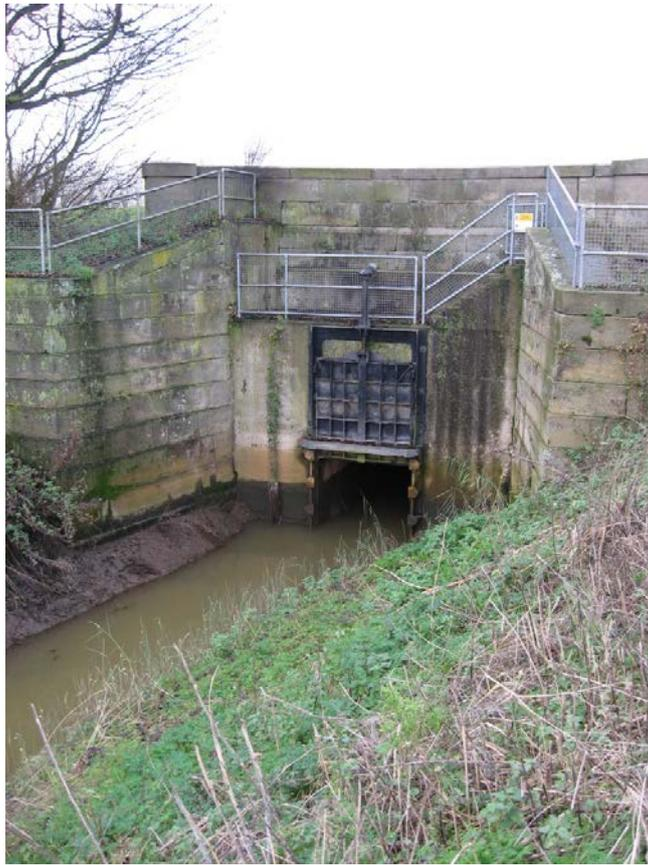
**Figure 3.5** View of flap valve (note valve is open)
