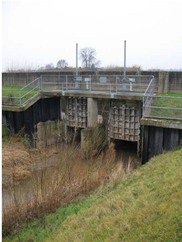
**Figure 3.19 View of flap valves – the Retarder controls the flap at bottom left**
