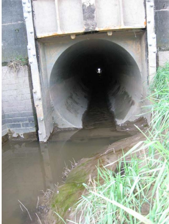
**Figure 3.10** View of ACE flap-valve with fish access flap (open)
