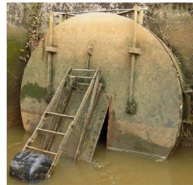
Self Regulating Tide-gate showing how the float allows a smaller flap to open as the tide rises
