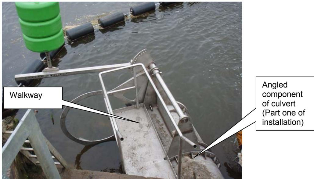
**Figure 3-11 Site specific adjustment to SRT at Lymington**
