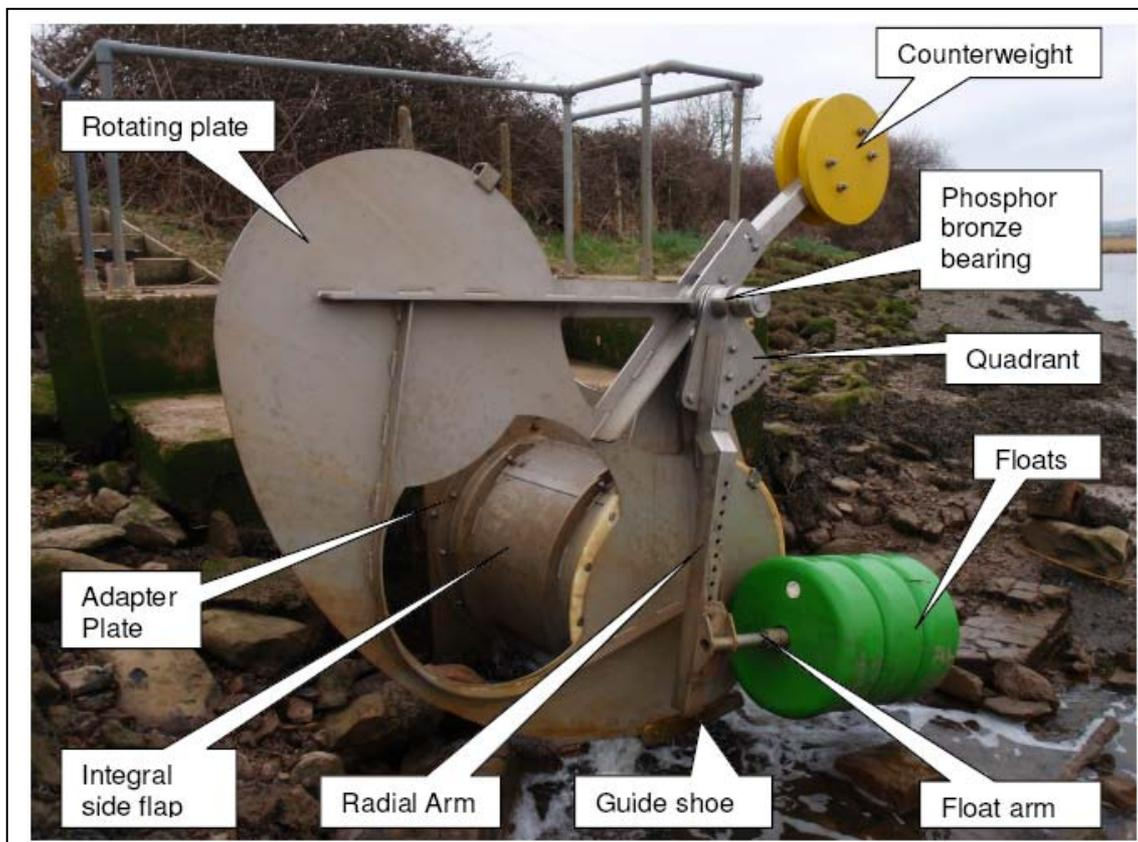
**Figure 2-1 Photograph of the Seaton gate showing key elements**
