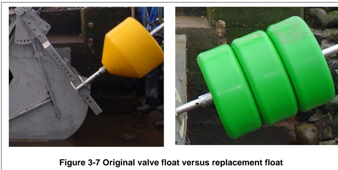
**Figure 3-7 Original valve float versus replacement float**
