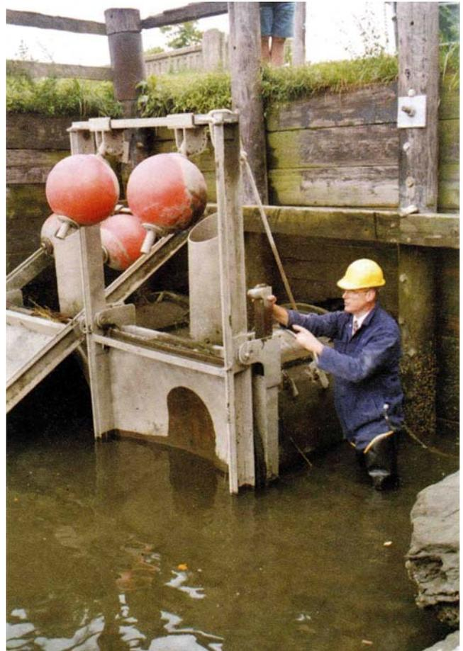
Self regulating tides gates have been extensively used to achieve regulated tidal exchange in the US, as here at Fairfield, Connecticut.
