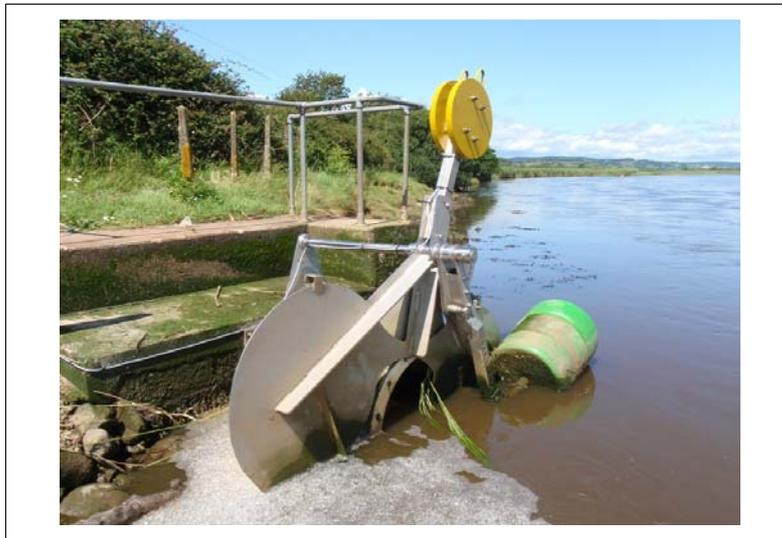
**Figure 3-6 SRT installation in partially open position enabling water passage. Here, water is shown draining out on a falling tide**
