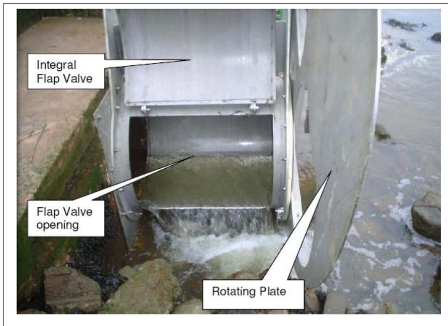
**Figure 3-8 Integral flap valve (shown held open manually)**
