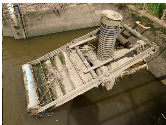
Figure 2: American design of floating flap SRT
