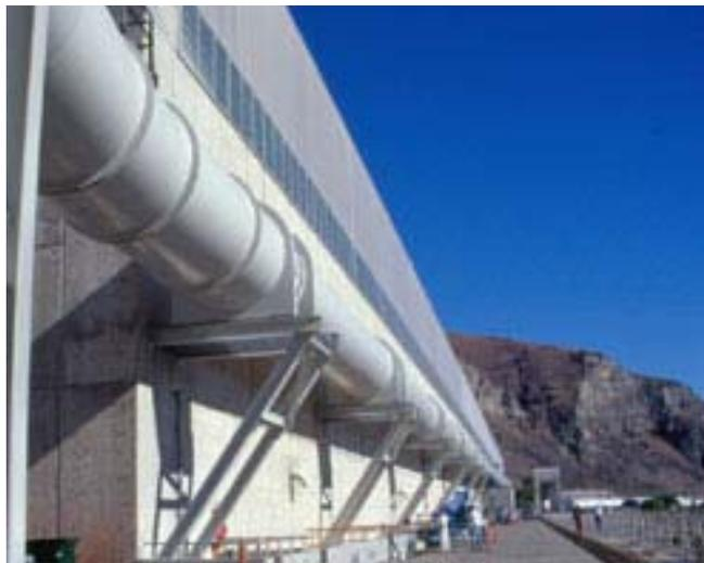
**Plate 3.15 The bypass pipe traversing the dam (Chelan County PUD).**
