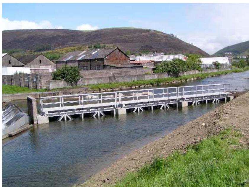
**Plate 3.1 Fixed panel screen installed on the R. Afan, Port Talbot in 2003, to prevent salmonid smolts from entering the docks feeder.**
