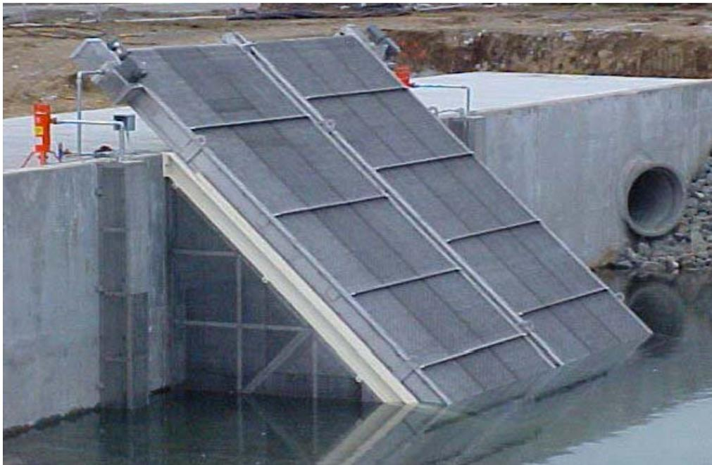
**Plate 3.10 Example of a self-cleaning belt screen installation. The screens are sealed at the sides to prevent fish or debris entrainment; screened weed and other debris are dumped on the ground below the top of the screen (courtesy of FPI Water Screens, USA: [www.fpi-co.com](http://www.fpi-co.com))**
