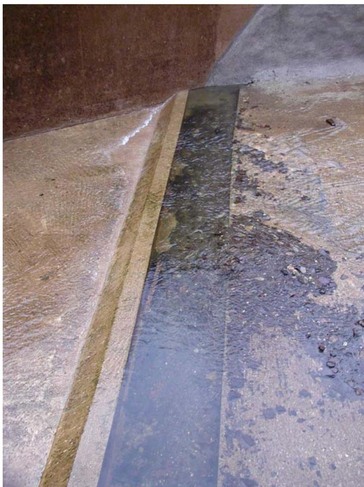
**Plate 3.15 Eel bypass trough at Backbarrow hydropower scheme, R. Leven, Cumbria (Spiby, 2004).**
