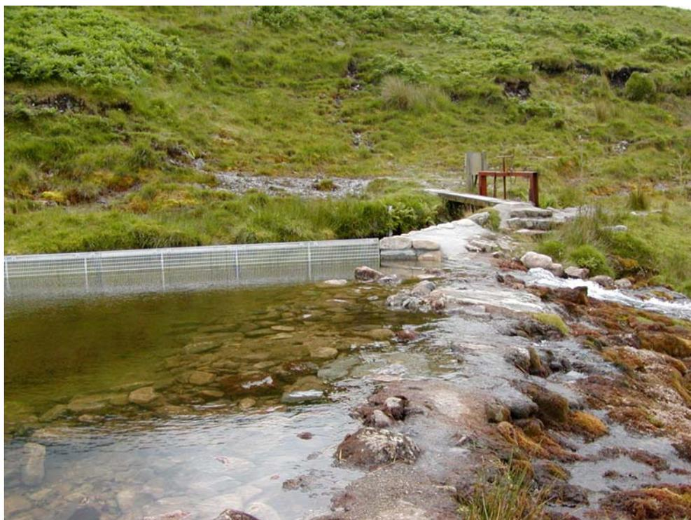
**Plate 3.2 Fixed panel screen installed on the R. Plym, Devon in 2003, protecting the entrance to an industrial supply offtake.**
