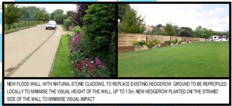
NEW FLOOD WALL, WITH NATURAL STONE CLADDING, TO REPLACE EXISTING HEDGEROW. GROUND TO BE REPROFILED LOCALLY TO MINIMISE THE VISUAL HEIGHT OF THE WALL, UP TO 1.5m. NEW HEDGEROW PLANTED ON 'THE STRAND' SIDE OF THE WALL TO MINIMISE VISUAL IMPACT
