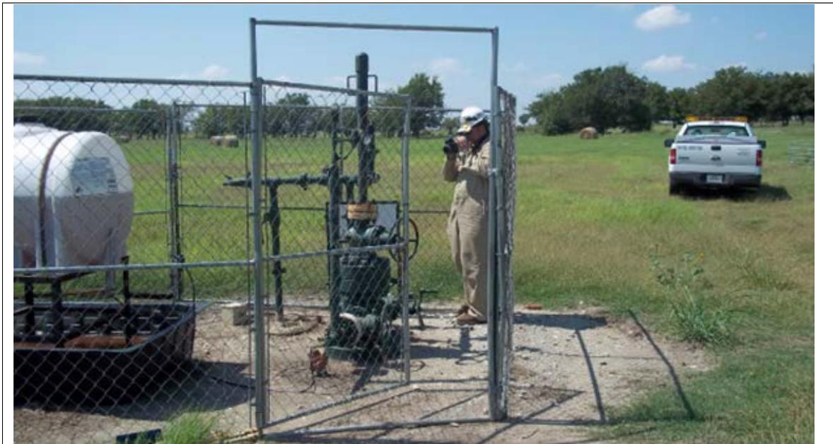
**Figure 5.5 Leak identification using a FLIR™ (IR) camera**
