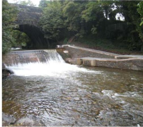
The Larinier-type Pass, with two flights of baffles and two rest pools, will allow salmon, sea trout and brown trout to travel to their preferred spawning areas. The Pass, which opened in early 2009, has been designed so that a fish counter can be installed, and this - along with monitoring the juvenile salmonid population upstream, and the catches anglers make – will help in judging just how successful it is.
