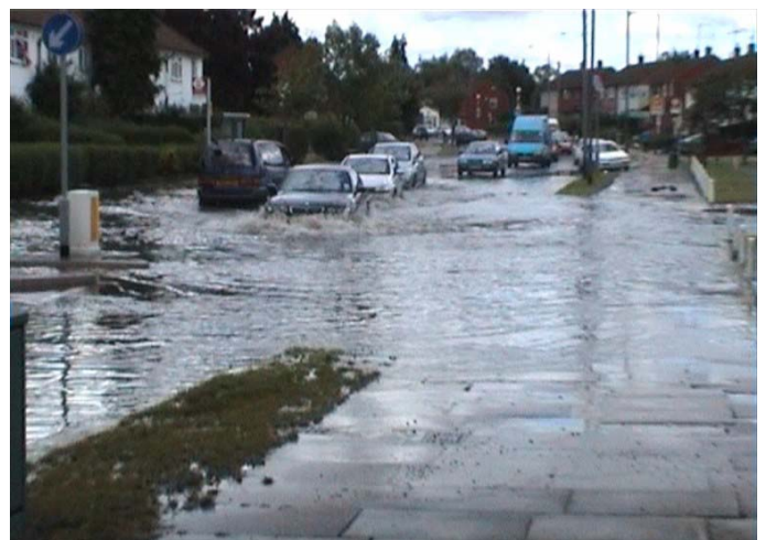
Flooding from multiple sources, courtesy of John Timms, MBE
