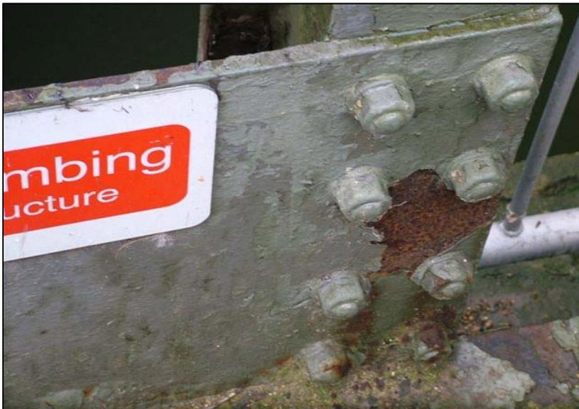
**Figure 4.16 Example of failed paint finish on the Great Ouse.**
