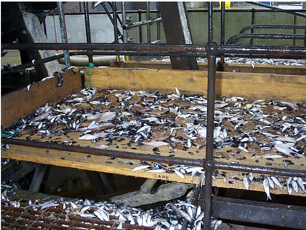
Figure 6-23 Fish that have overshot the hopper collecting on a scaffold boards inside a drum screen chamber
