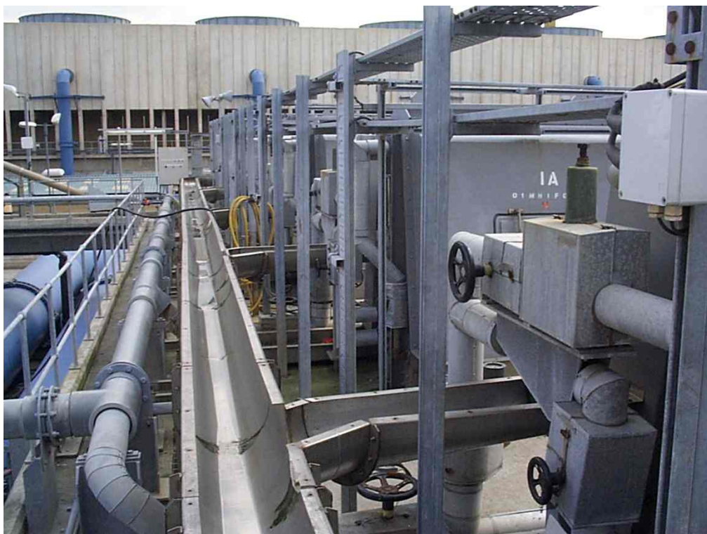
Figure 6-20 Example of fish return launders. Launderers should be covered to reduce predation risk. Larger radius (3 m) swept bends reduce the risk of debris and fish becoming caught in bends.
