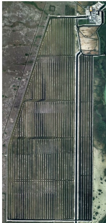
Figure 3-2 Aerial view of Turkey Point cooling canals
