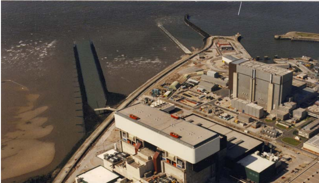
Figure 4-9 Inshore outfall structures for Heysham A and Heysham B
