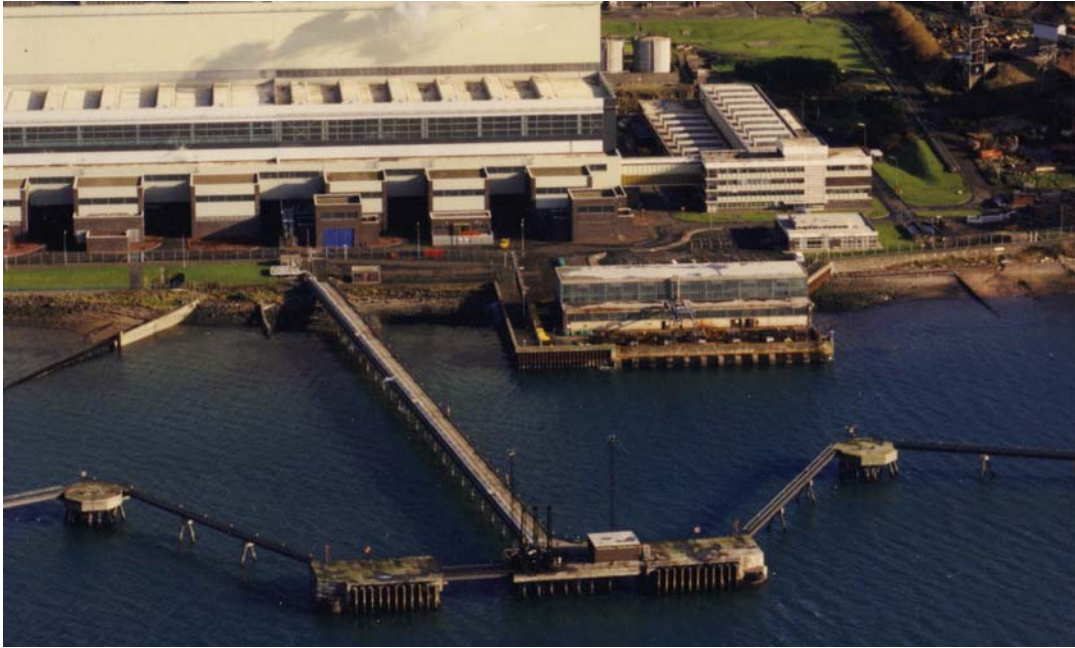
Figure 4-2 Inshore Intake at Ballylumford B, Larne
