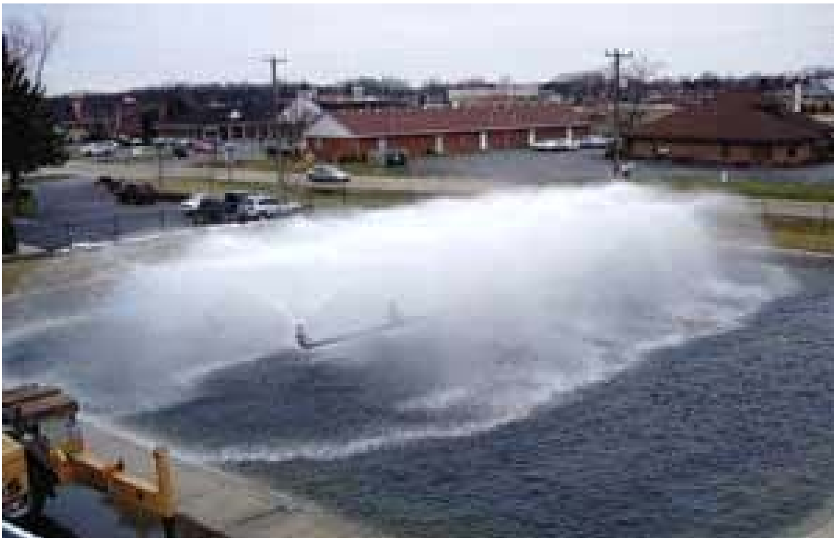
Figure 3-3 Spray cooling (photo courtesy Siemens Power Generation)
