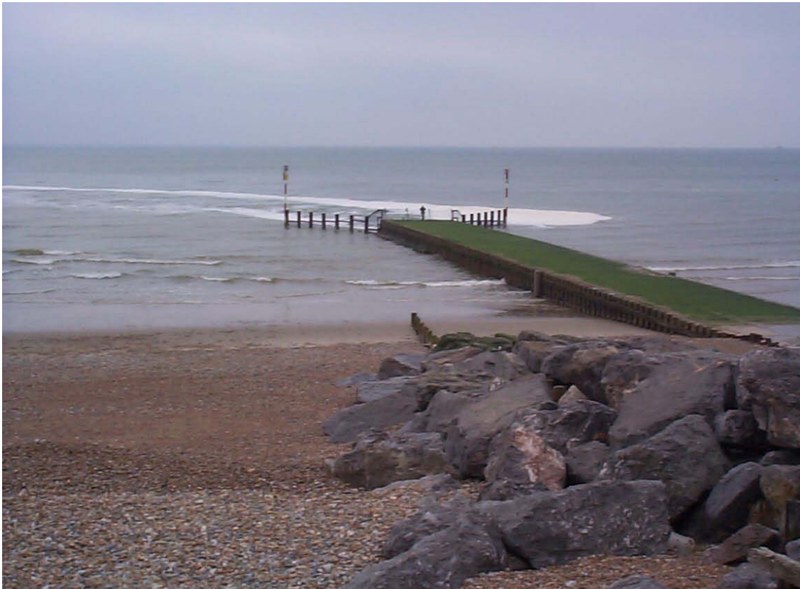
Figure 6-24 A thermal plume, made visible by alginate-induced foaming
