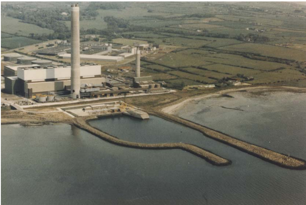
Figure 4-3 Inshore Intake at Kilroot, Carrickfergus
