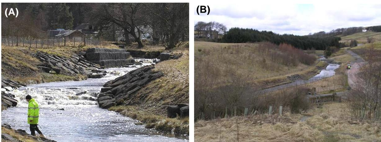
**Figure 6. Use of gabions to stabilise banks of the River Nent, Cumbria (A) and re-grading, capping and vegetation of spoil material along the same stretch of river (B)**
