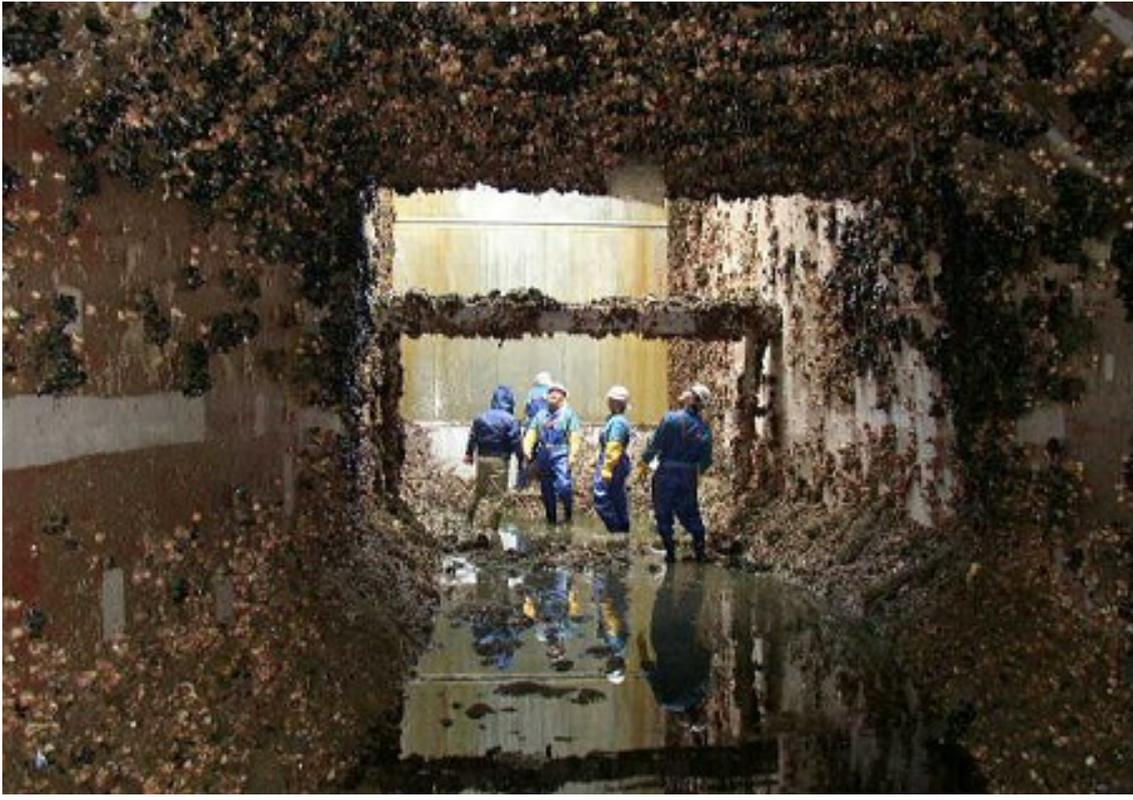
**Figure 4.3 Mussel infestation in a main cooling water culvert (drained for maintenance) (By permission of KEMA)**
