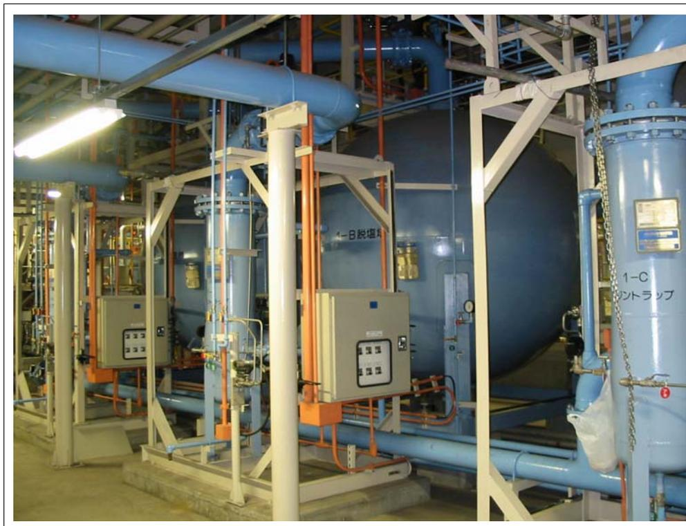
**Figure 6.1 Standard deep bed condensate polishing plant (resin vessels) in a fossil fuel power station – similar systems are used in many PWR power plants (see Section 1.6.3) (By permission of Graver Water Systems LLC)**
