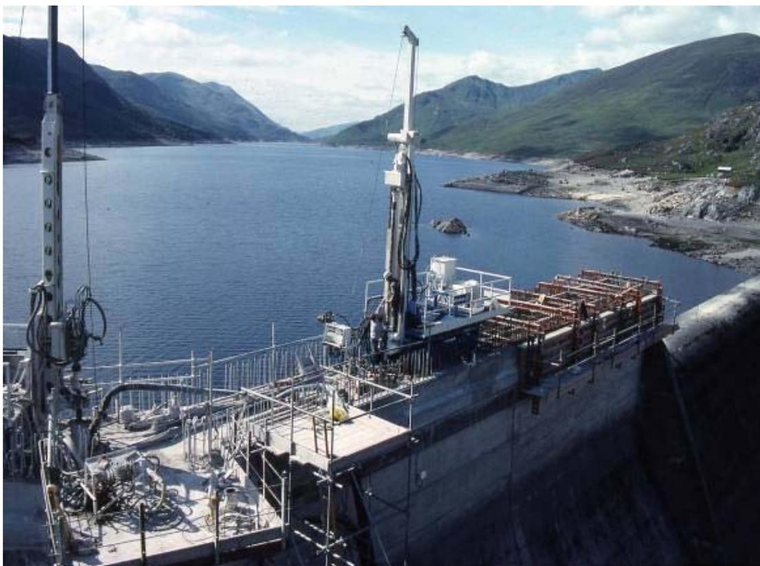
Figure 5-28 Post-tensioning works at Mullardoch dam
