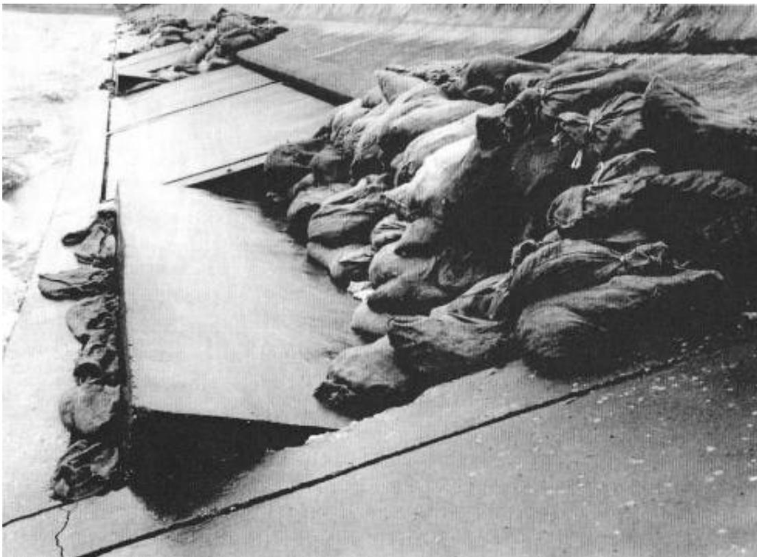
Figure 5-21 Section and damage to the upstream protection at Blithfield dam (after Herbert *et al.*, 1995)
