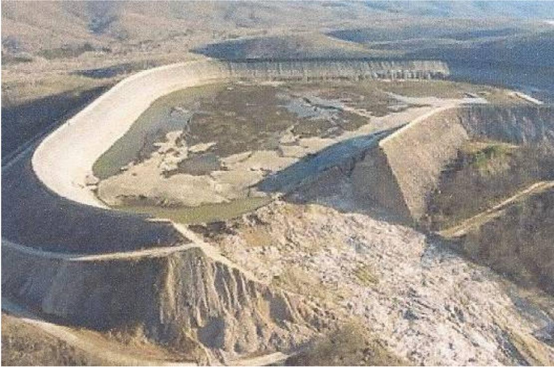
**Figure 5-32 Breach through Taum Sauk embankment**
