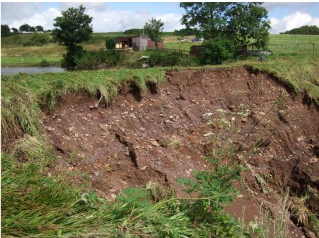
**Figure 5-20 Erosion of the downstream shoulder fill due to overtopping at Maich Water**
