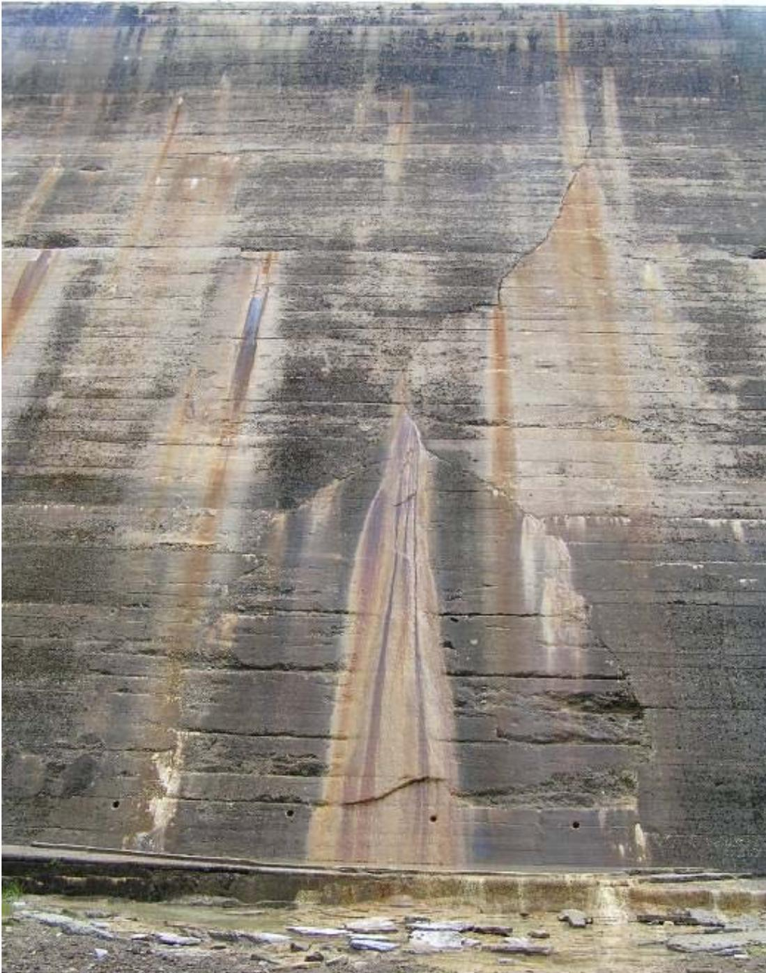
**Figure 5-22 Vertical cracks in Blackwater dam**
