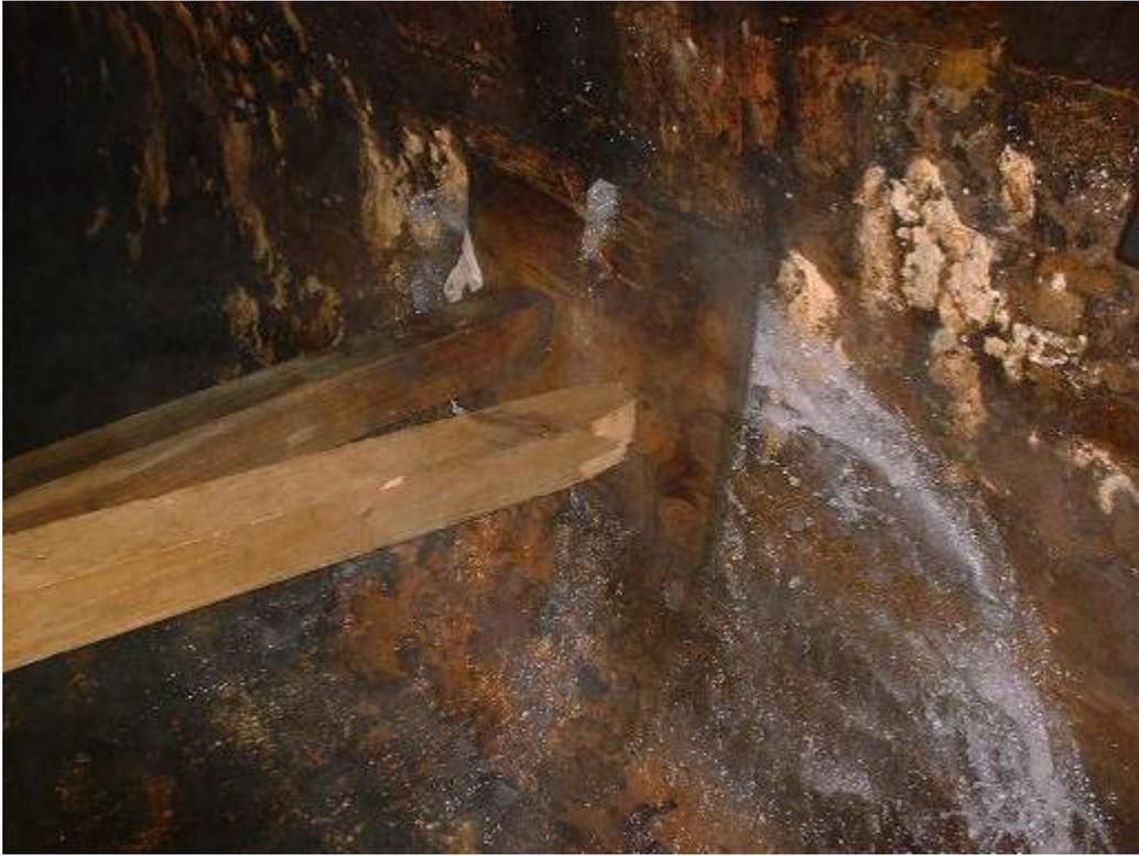
**Figure 5-11 Leakage in the draw-off culvert at Yarrow embankment and temporary plug (after Gardiner *et al.*, 2004)**
