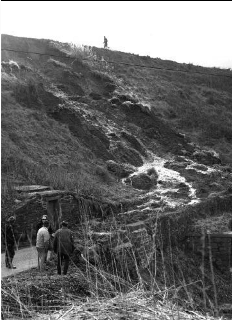
**Figure 5-17 The downstream slip at Combs dam (after Dutton, 2001)**
