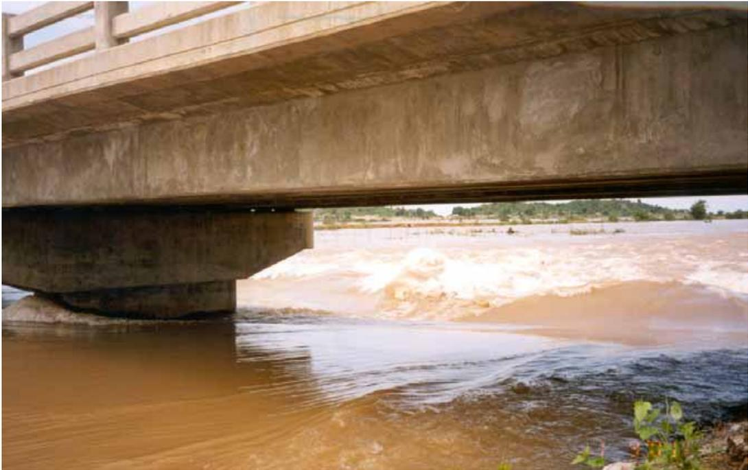
**Plate 2 – Supercritical flow through bridge – Cambodia**
