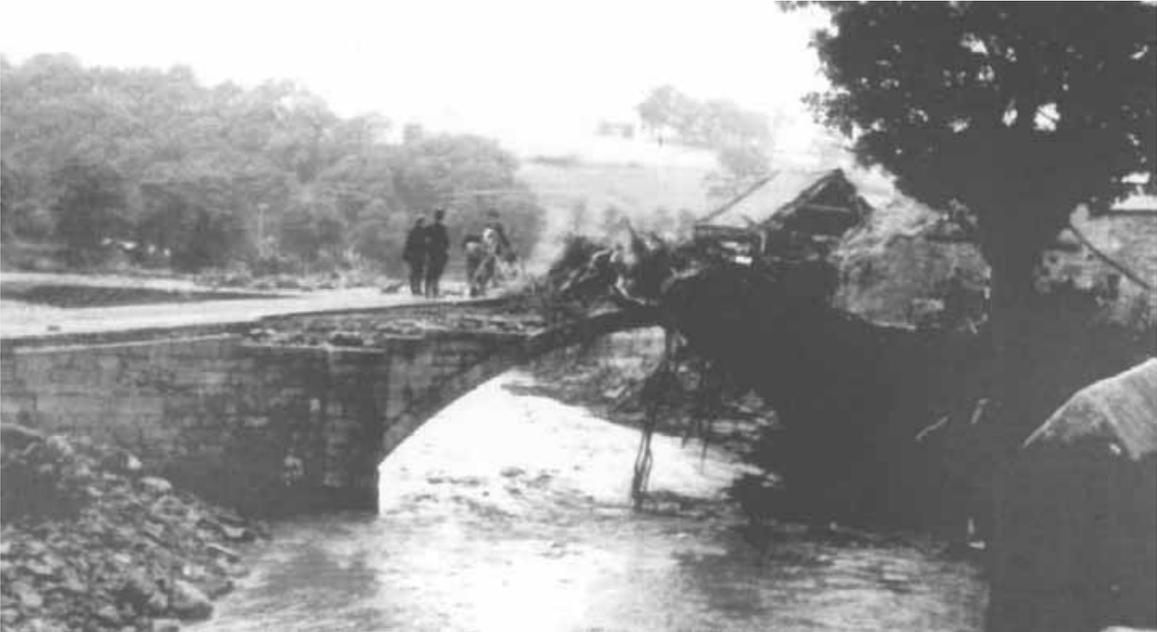
**Figure 16: Results of a catastrophic flood through a single arch bridge in Yorkshire.**
