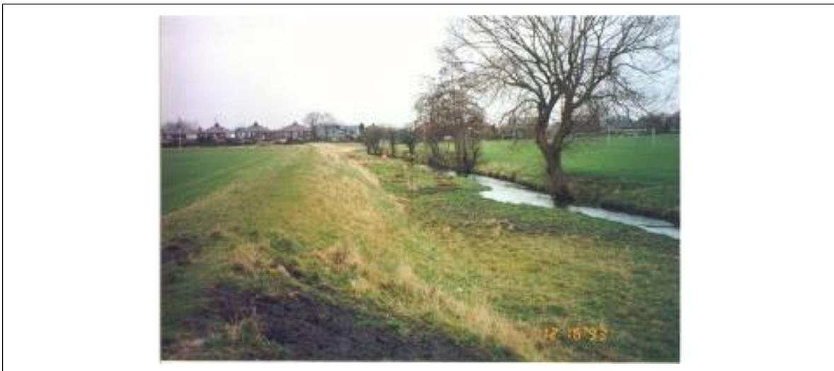
**Figure 6.15 Example of narrow low-flow channel close to Warrington**
