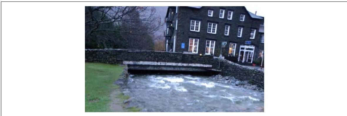
**Figure 6.2 Example of limited capacity of a bridge due to sediment deposition (water depth about 30 cm)**
