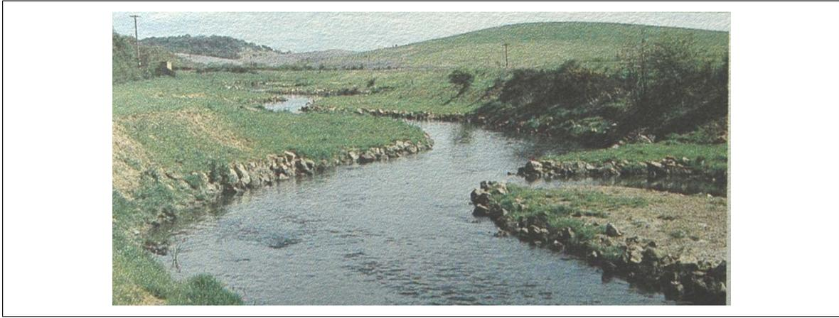
**Figure 5.4 Channel narrowed by rock revetment**
