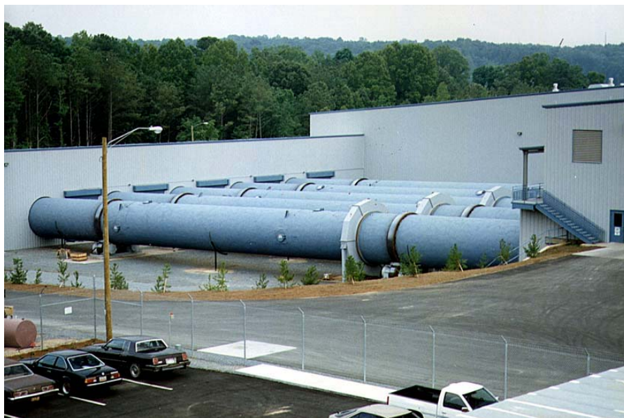
Figure 10-8: Bedminster composting system – rotating drums
