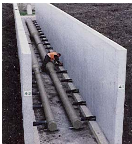
Figure 10-32: VAR composting system – aeration system between bays
