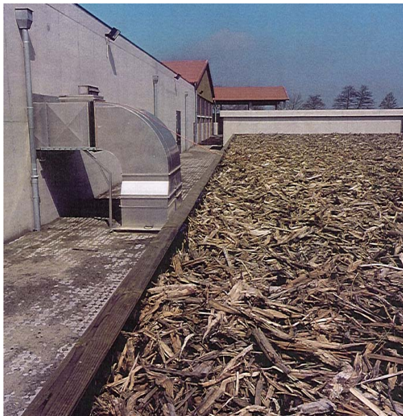
Figure 10-41: External biofilter and ducting taking exhaust gases from tunnels
