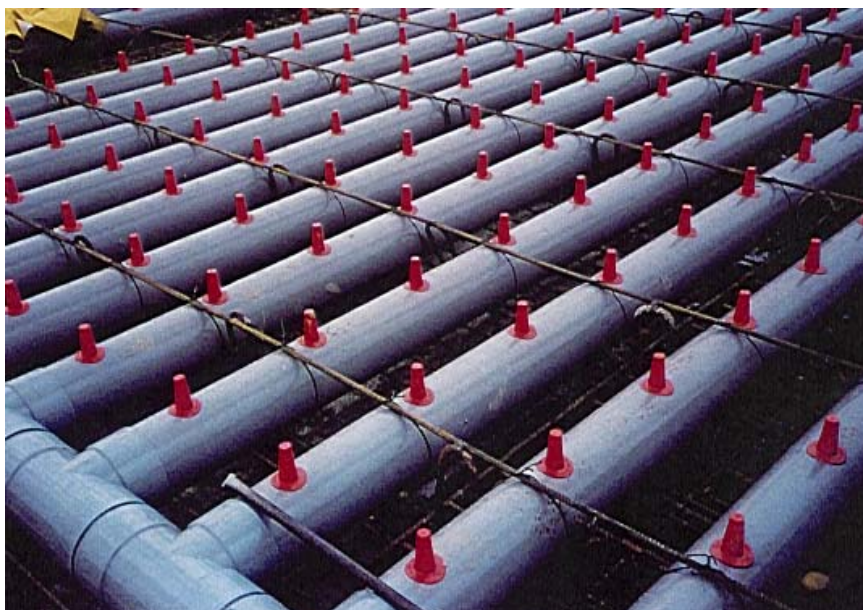
Figure 10-40: Aeration pipes in tunnel floor during construction showing spigots
