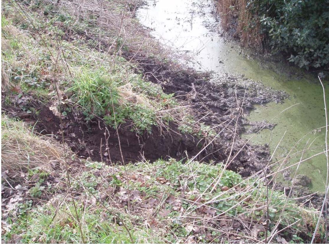
3. Showing clogged up ditch. Holding the water back will reduce water flow to Catfield Fen. Conclusion: clean out ditch
