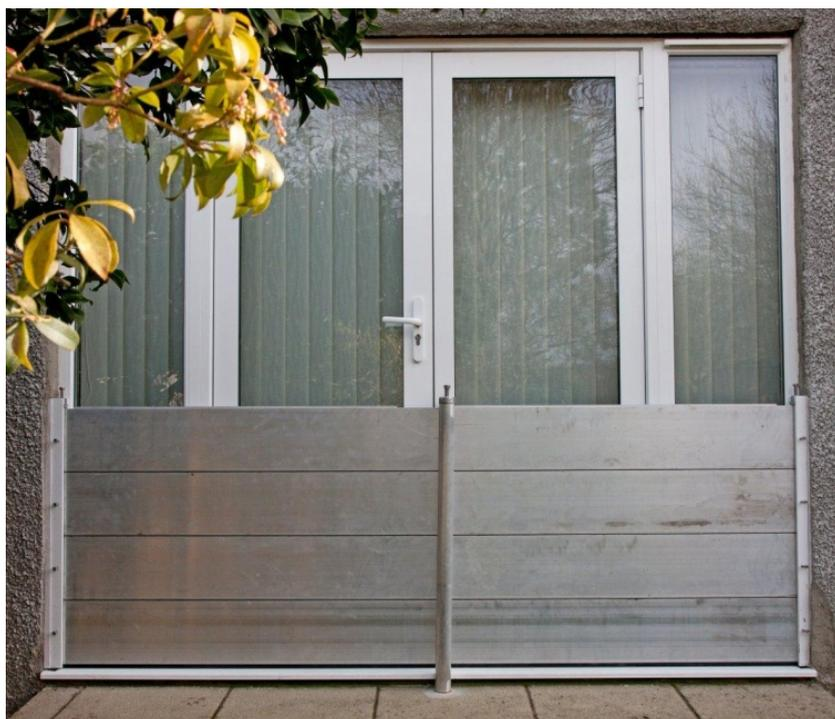
Implemented property-level protection – water-tight door panels coupled with sealable air brick
