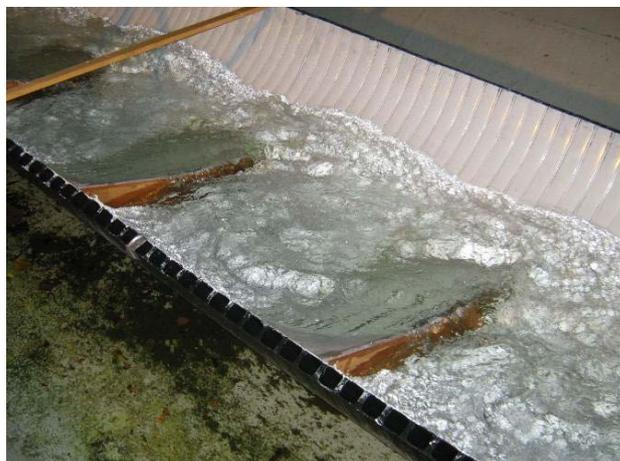
**Culvert with baffles to improve eel passage**
