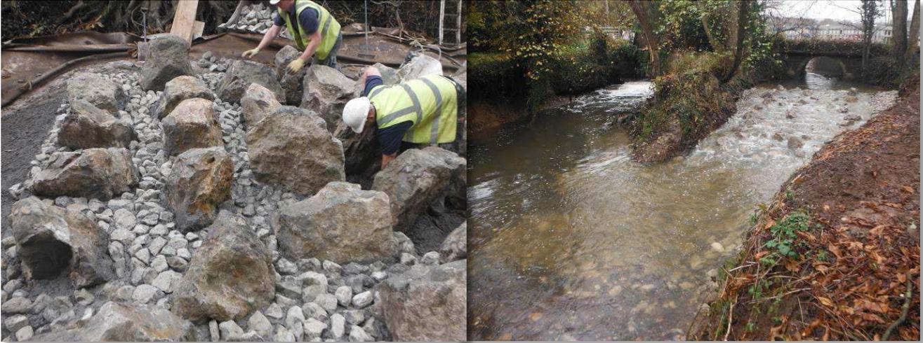
**LEFT: Smaller rocks being placed by hand into the concrete surface of the rock ramp at Sharpsbridge. RIGHT: Completed rock ramp including downstream rock toe.**
