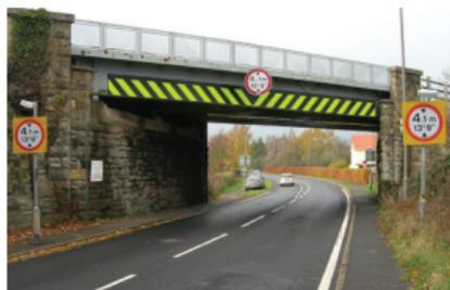
*Warning chevrons and mandatory roundel signs showing the limit on vehicle height at a flat soffit bridge*
