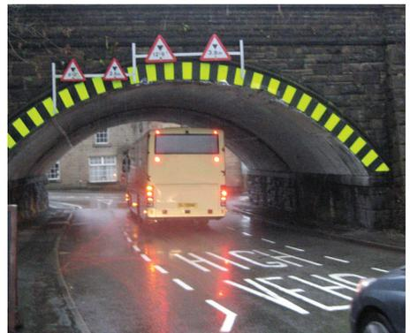
White lines on the road and 'goal posts' on the arch indicating the extent of the signed vehicle height limit
