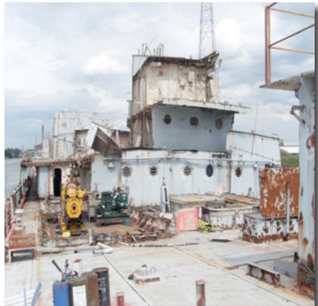
Dismantling forward structure removed up to the funnel
