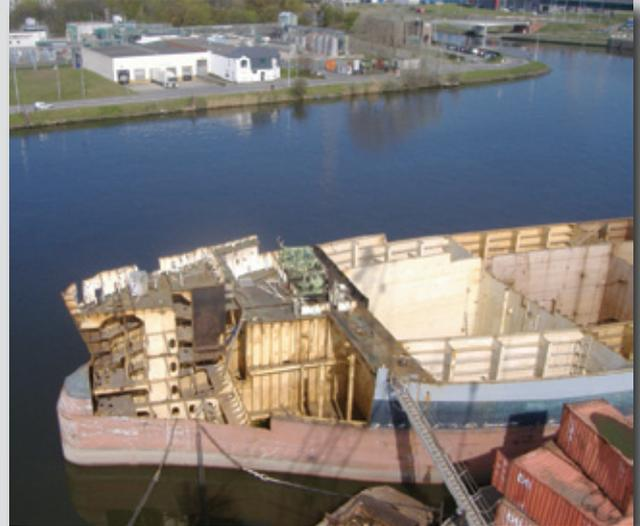
showing the stages of pre-cutting, ready for the hull to be towed up the slipway
