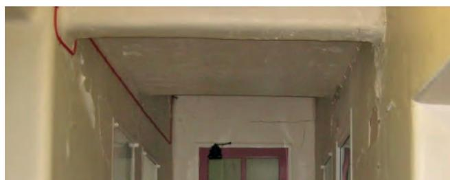
Internal walls painted surface-Condition Grade C - Poor; flaking and peeling emulsion finish.
