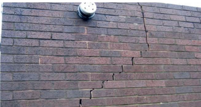
Condition Grade C - Poor; structural cracking, leaning, within brickwork structure.
