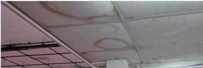
Condition Grade C - Poor; damp stained tiles, distortion to grid.
