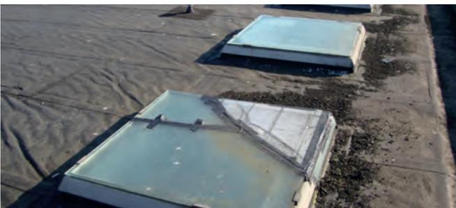
Condition Grade C - Poor; cracked and bubbled covering, deteriorated flashing details.
