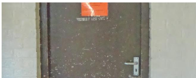
Internal door painted surface-Condition Grade C - Poor; flaking and worn painted finish
