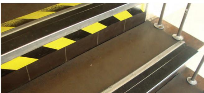
Condition Grade C - Poor; wear to surface, nosings loose or missing.
