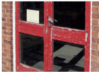
Condition Grade C - Poor; aged deteriorated timber doors (note decorations separately considered)
