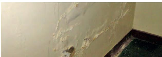
Condition Grade C - Poor; damp affected and 'blown' plasterwork
