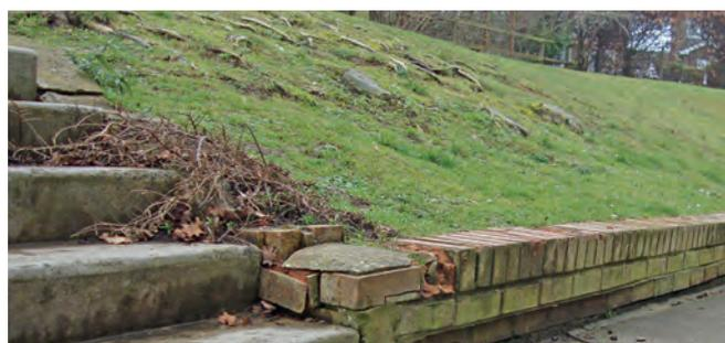
Condition Grade C - Poor; spoiled brickwork retaining wall.
