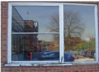
Condition Grade C - Poor; wet rot affected timber frame
