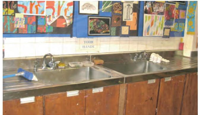
Condition Grade C - Poor; aged, damaged and broken fixed cupboard units
