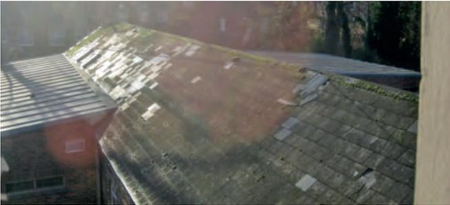
Condition Grade C - Poor; extensive slipped and missing slates.
