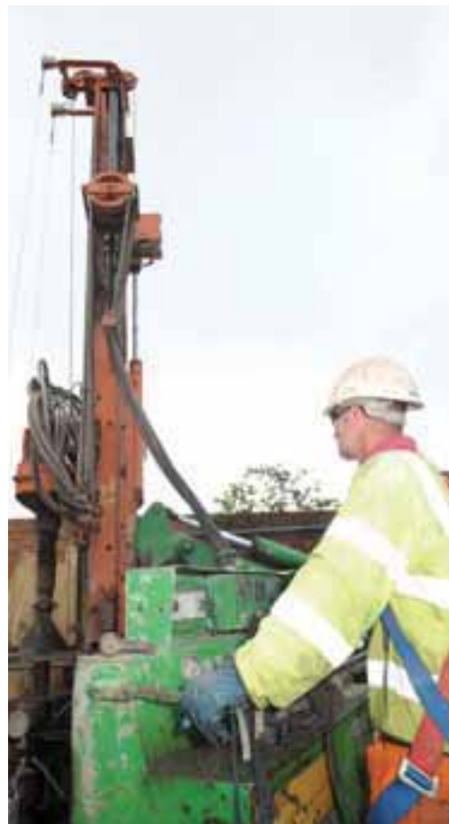
Grouting a coal mine shaft
