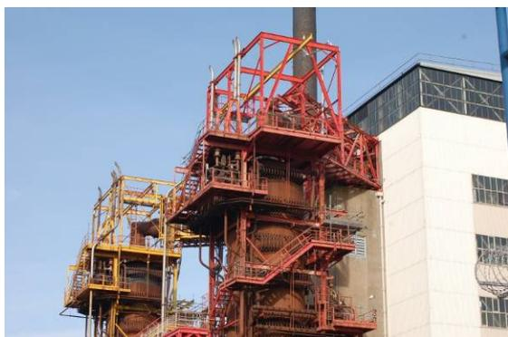
In March 2010, work to strip asbestos cladding from the heat exchangers, turbine halls and associated plant at Calder Hall was completed. The project, which has taken over five years, has seen the removal of 2,300 tonnes of asbestos cladding under extremely difficult working conditions and is considered to be the largest of its kind in Europe. Furthermore, this deteriorating asbestos insulation presented the highest conventional safety hazard across the NDA estate.
