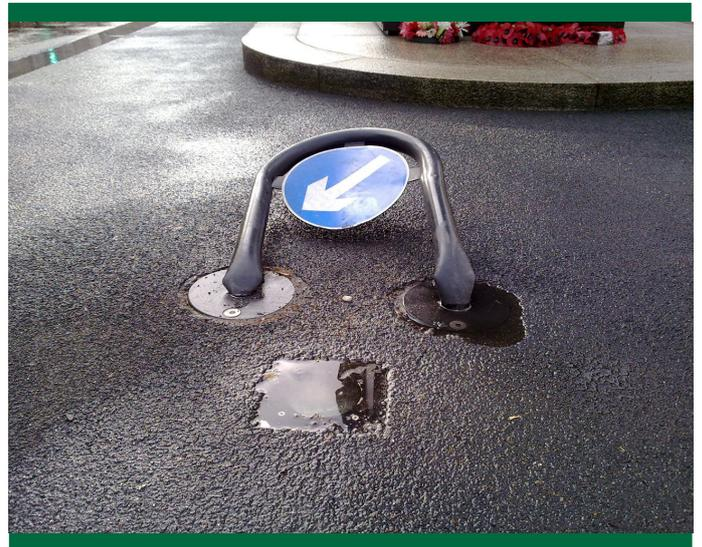
Figure 8: Damaged hoop mounted sign
