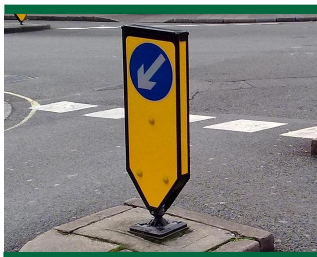
Figure 6: Retroreflective self-righting bollard
