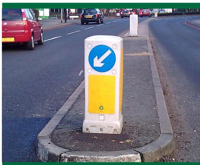
Figure 5: Mains powered internally illuminated traffic bollard
