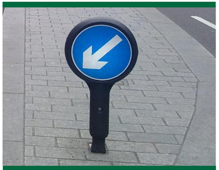
Figure 10: Low level sign on deformable posts
