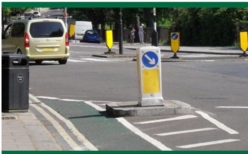
*Figure 15: Cycle gap with an inappropriate keep right sign*
