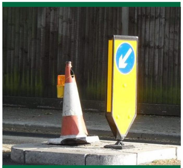
Figure 18: Check damaged equipment is still necessary before replacing
