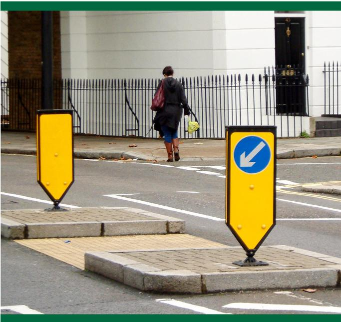
Figure 16: RSRBs with retroreflecting material on the rear faces
