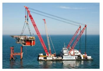
extensions and placement of the abrasive cutting tool into each of the legs for cutting. Each leg was cut at least 3m below the natural seabed. As each leg was cut a rigging arrangement was attached to the top of the jacket allowing the HLV to lift the jacket clear of the seabed immediately
