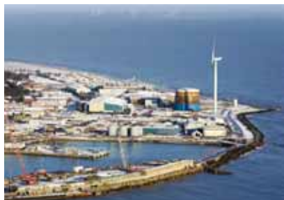
Above top: Scour pits around the monopiles at Scroby Sands, off the Norfolk coast Above: Lowestoft harbour, with Scroby Sands wind farm in the distance Right: Catch being hauled aboard a commercial vessel
