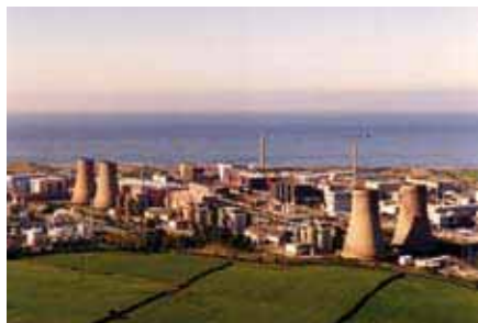
▼ British Nuclear Group Reprocessing plant (THORP) at Sellafield
