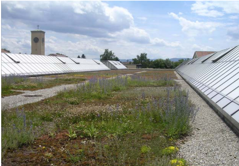
Figure 2. Typical extensive green roof (courtesy of Green Roof Consultancy)
