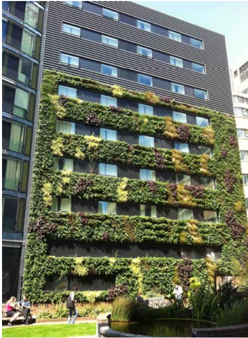
Figure 4. Living wall installation at Tower Gateway (courtesy of Gary Grant)
