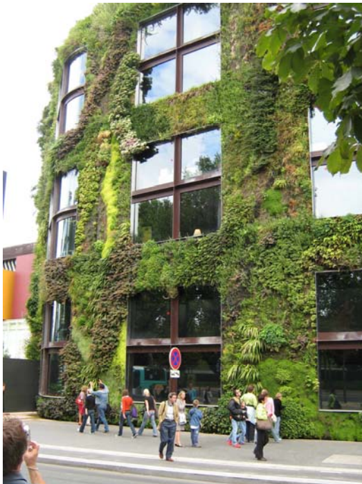
Figure 5. Living wall installation, Paris (courtesy of Gary Grant)
