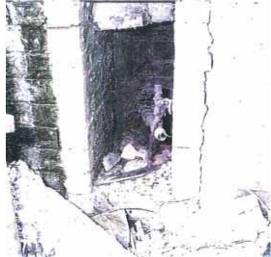
Figure 24 – The LPG underground pipeline enters the building in an alcove in the basement
