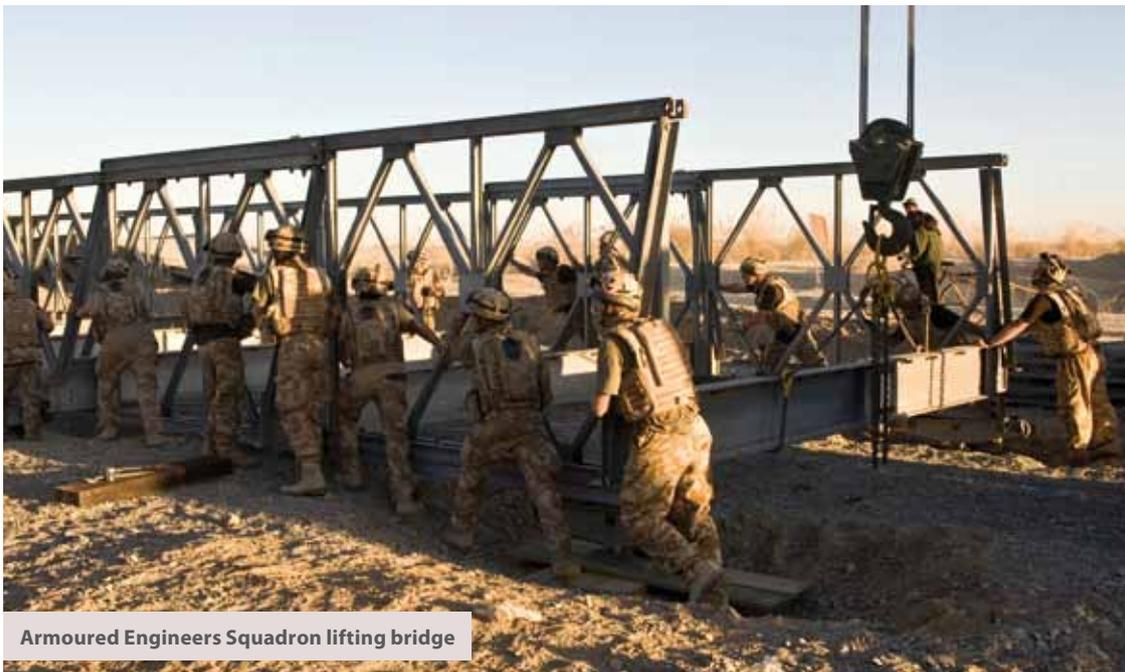
Armoured Engineers Squadron lifting bridge
