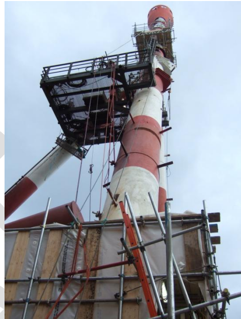
MCP-01 - Flare ready for heavy lift
