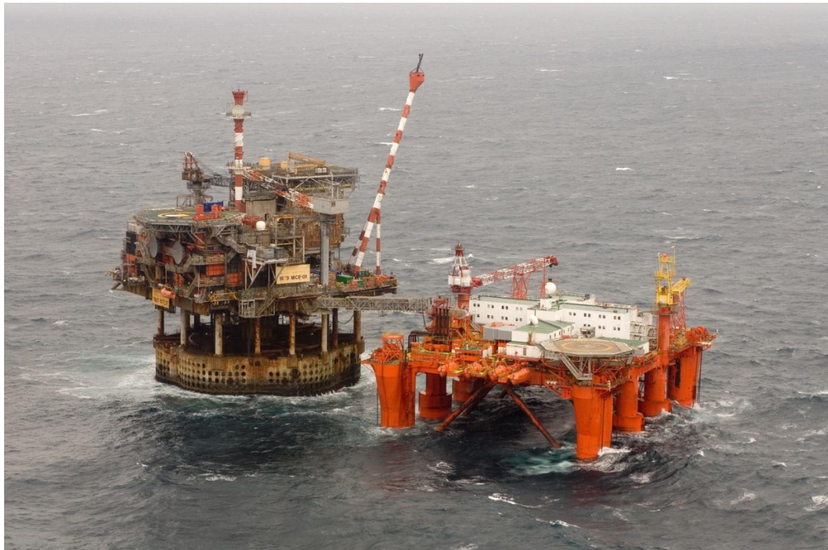
2006 at start of topsides removal – flotel “Port Reval” in attendance
