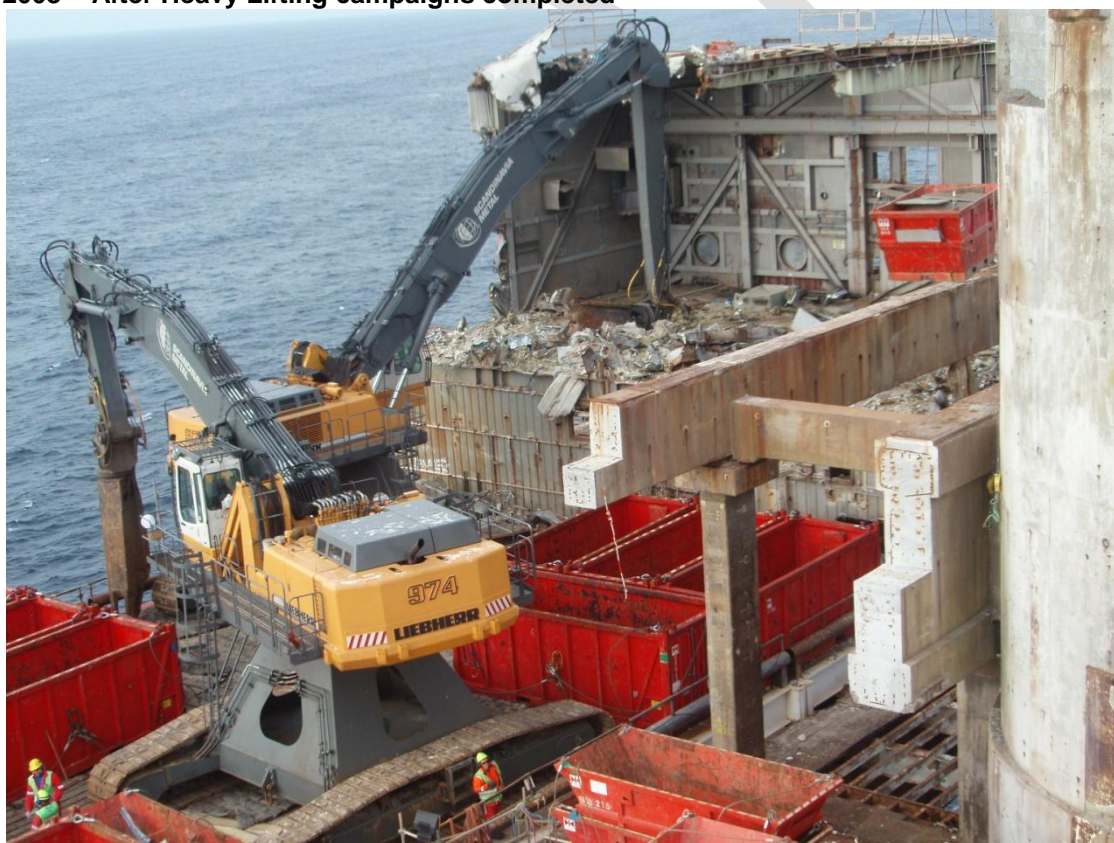
Large Demolition Excavators dismantling Turbine Hall
