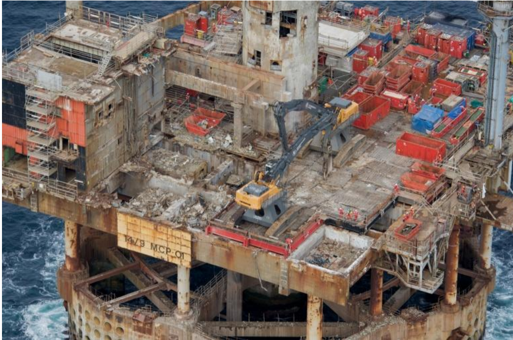
MCP-01 - Piece Small Demolition in progress with excavators
