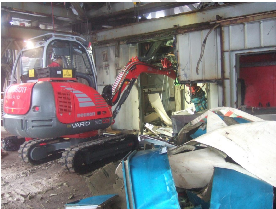
Demolition Excavator processing architecture and fittings
