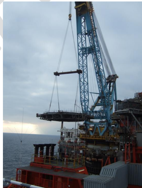
MCP-01 - 3 piece helideck as single lift 1
