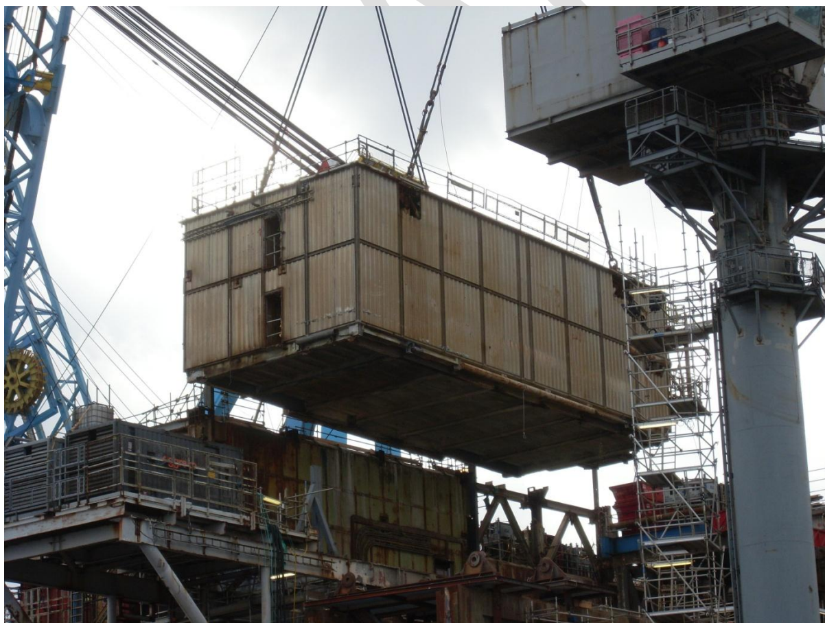
2008 – Removal of PLQ ( Quarters) module
