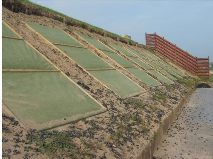
7. The fire at Strensall was in part at least caused by tracer in treated timber. Timber is being used more and more on ranges to minimise the need for grass cutting. At Strensall the timber was placed over granulate at the top of the stop butt; this allowed air to flow up under the timber that was engaged with tracer ammunition. Had the timber been set into earth or sand the outcome might not have been so drastic.
