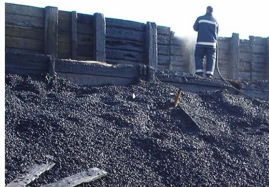
8. Heavy use ranges with large volumes of granulate and particularly those where tracer is fired should ensure that orders for the range warden include checking granulate after each days firing and if there is any sign of latent heat in the rubber, dowse with water. This precaution includes barrack ranges with granulated rubber bullet traps as well.
