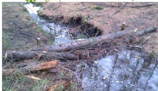
One of >150 large woody debris dams constructed in woodland streams to 'slow the flow'
