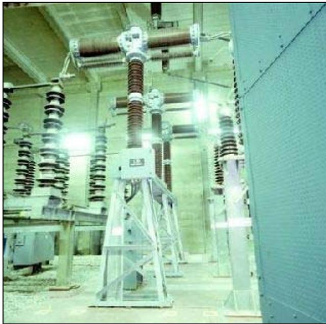
Figure A1-6: Indoor 275kV AIS circuit breaker
