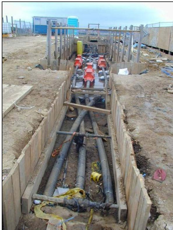
Figure A1-19: Underground Cable Joint Trench
