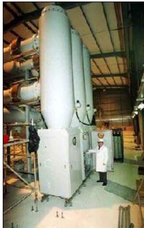
Figure A1-4: Indoor GIS circuit breaker
