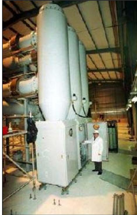
Figure A1-4: Indoor GIS circuit breaker
