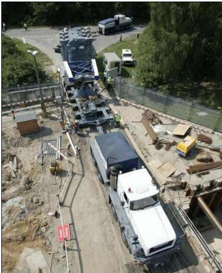
Figure A1-10: Delivery of an 1100MVA Transformer to Site
