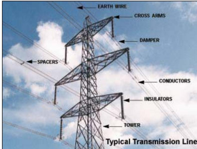
Figure A1-27: The Main Features of a Transmission Line
