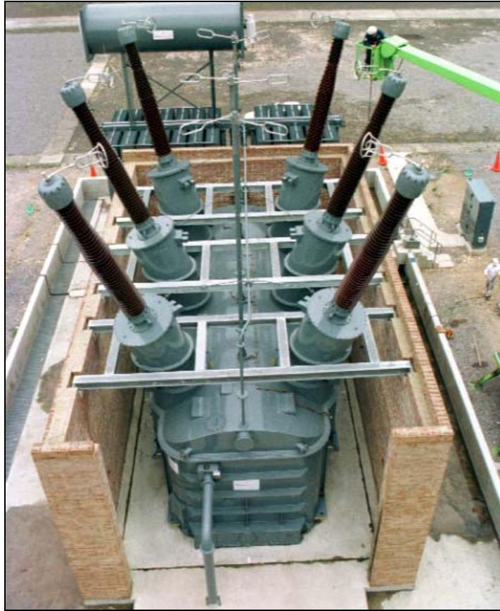
Figure A1-11: Typical Transformer being Installed within a Noise Enclosure
