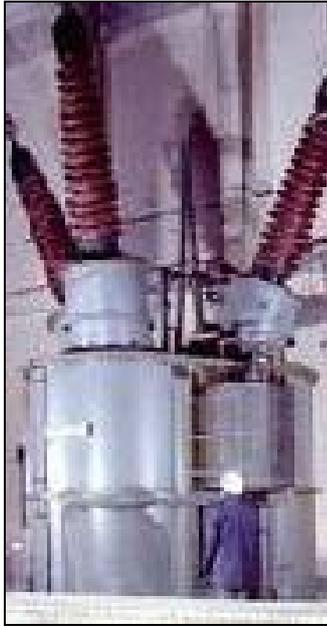
Figure A1-12: Inductive Reactive Compensator
