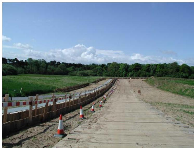
Figure A1-22: Access Swathe for Underground Cable Installation
