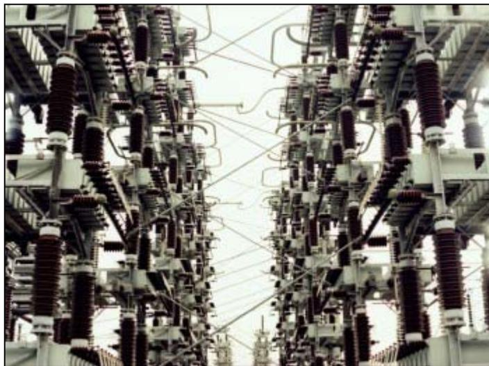
Figure A1-13: A Capacitive Reactive Compensator
