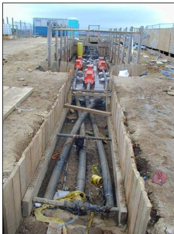
Figure A1-19: Underground Cable Joint Trench
