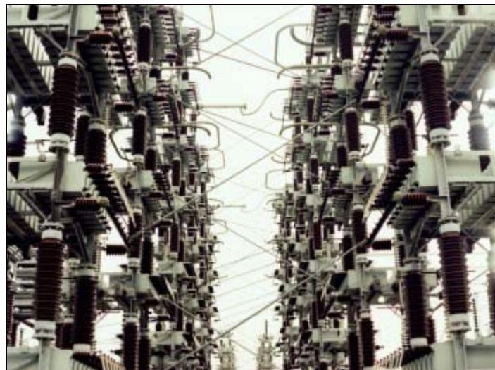
Figure A1-13: A Capacitive Reactive Compensator
