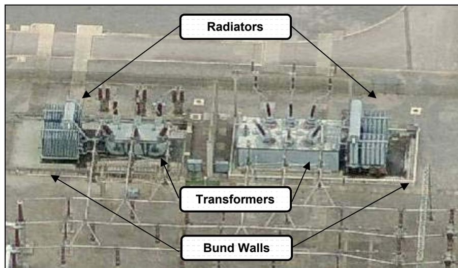
Figure A1-9: Typical 1100MVA Transformer Installation
