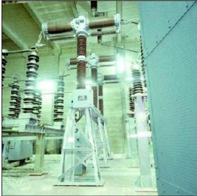
Figure A1-6: Indoor 275kV AIS circuit breaker
