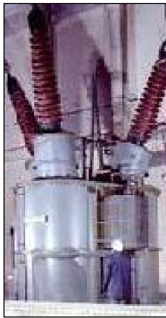
Figure A1-12: Inductive Reactive Compensator
