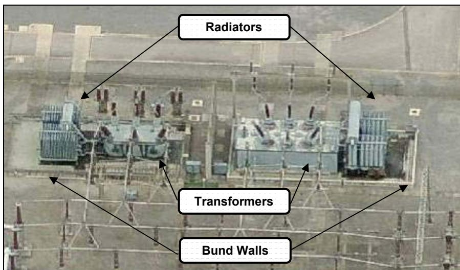
Figure A1-9: Typical 1100MVA Transformer Installation
