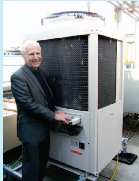
Energy Manager Harry Crofts and the IT Chiller
