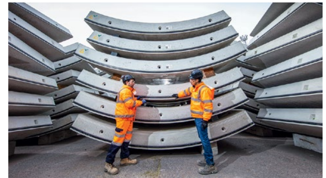
Engineers standing next to pre-cast concrete shapes prepared for the Thames Valley viaduct.
