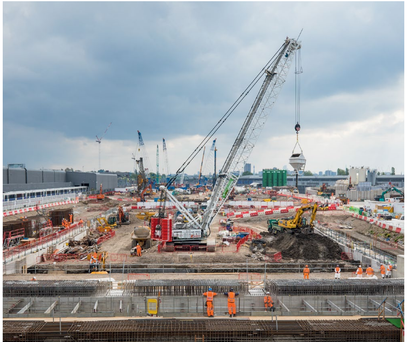
Construction work at Old Oak Common station.
