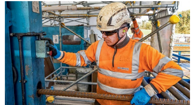
An engineer preparing rebar on-site.
