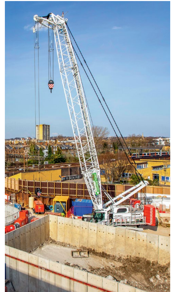
An electric crawler crane at Canterbury Road vent shaft.
