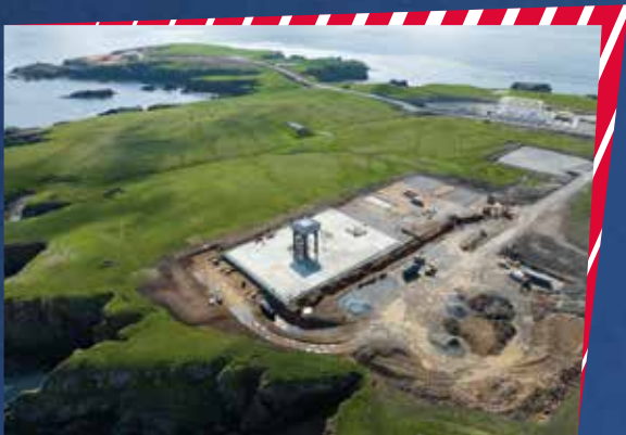
Completed launch stool and under-construction integration hangar at SaxaVord Spaceport.
