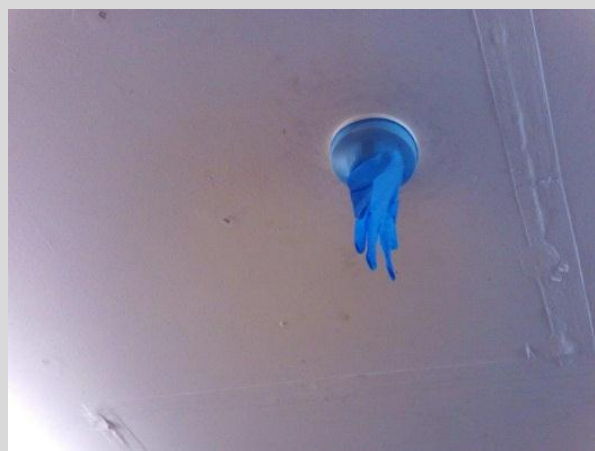
Picture 3- Smoke detection device covered by glove
