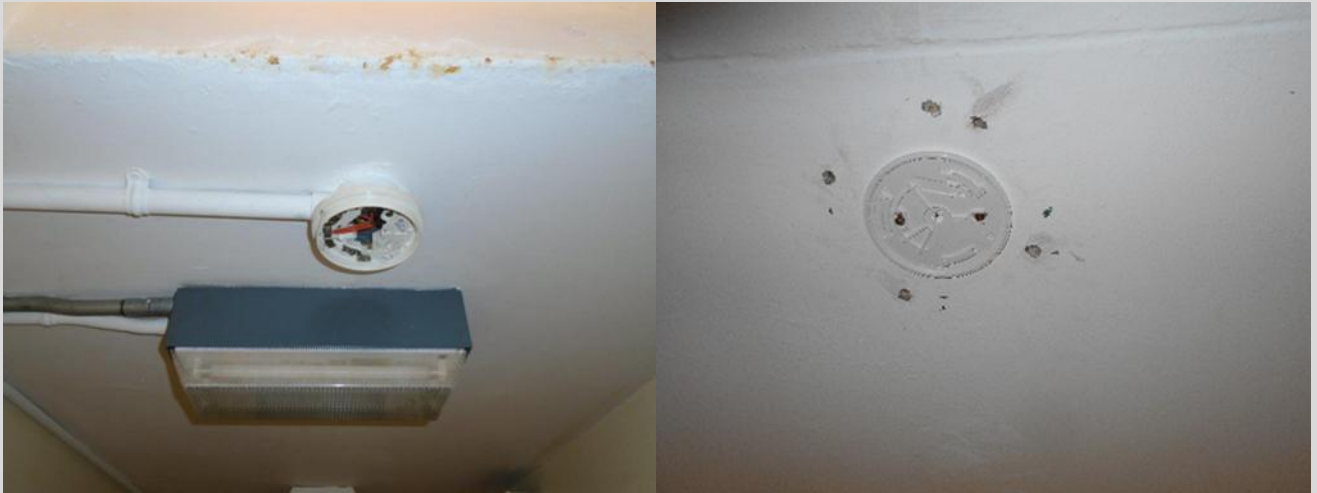
Picture set 4- Smoke detection devices missing from their mounting bases
